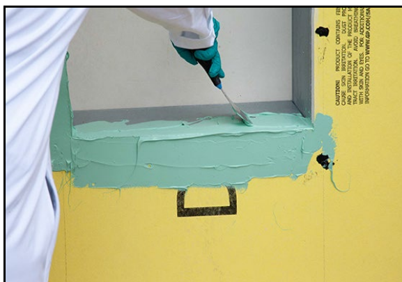
Figure 1: Application of DOWSIL™ 778 Silicone Liquid Flashing.
